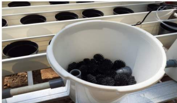
Fig 2:- Filter basket containing jagged rubber balls
