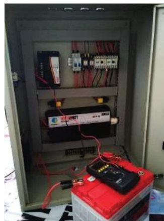
Fig. 9. PV Control System.
